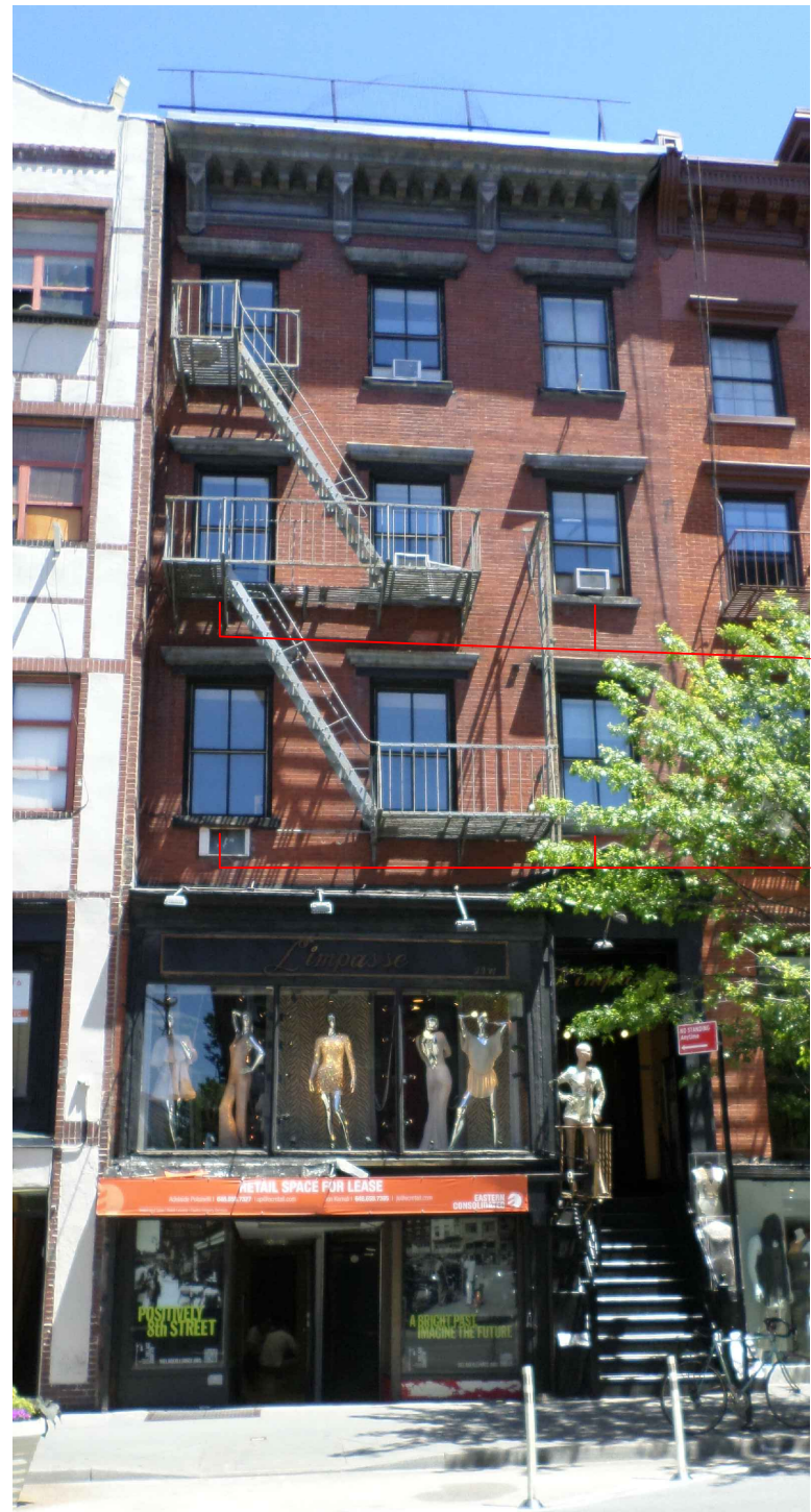
EXISTING FRONT FACADE
